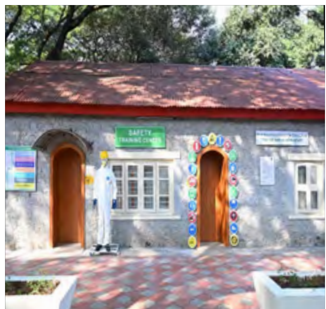
Safety Training Centre – A new State-of-the-Art Safety Training Facility at Kirloskarvadi
