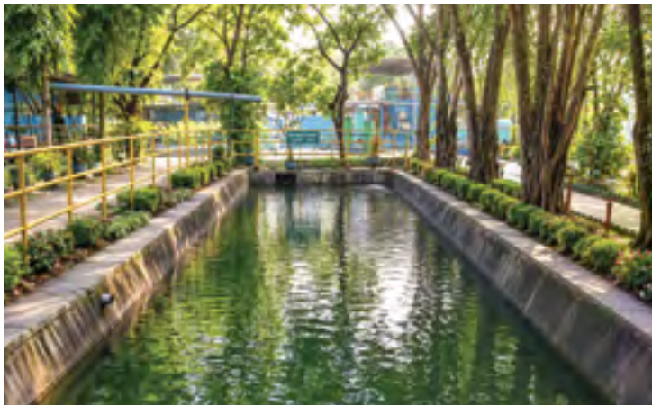
Water Recycling at Dewas Plant
